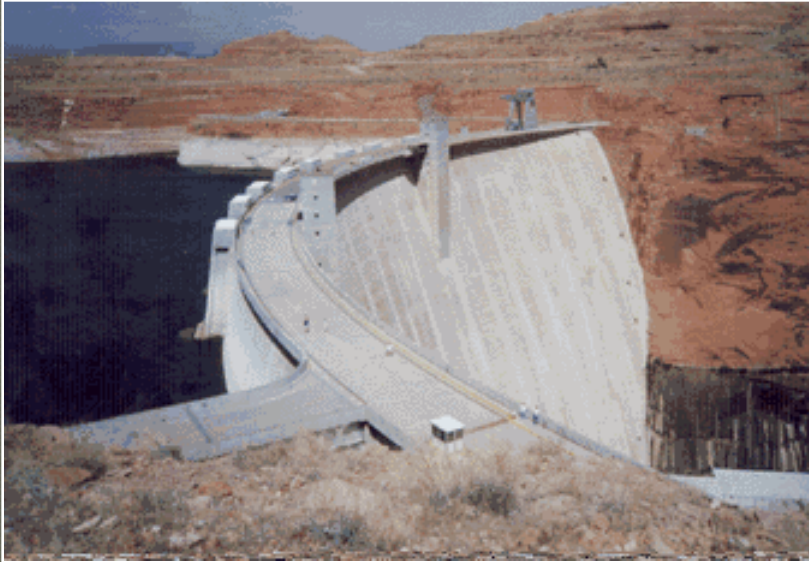
Glen Canyon Dam
